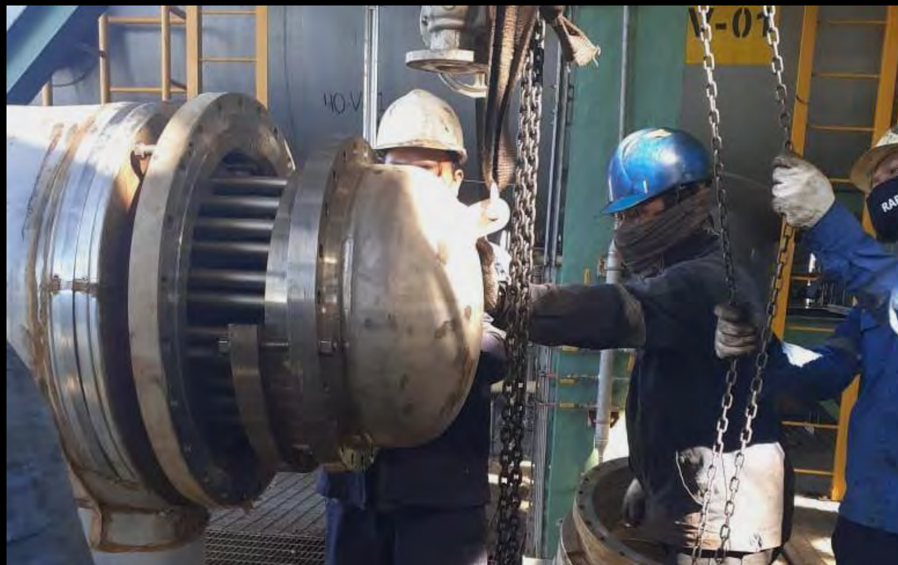
HEAT EXCHANGER DISASSAMBLING
