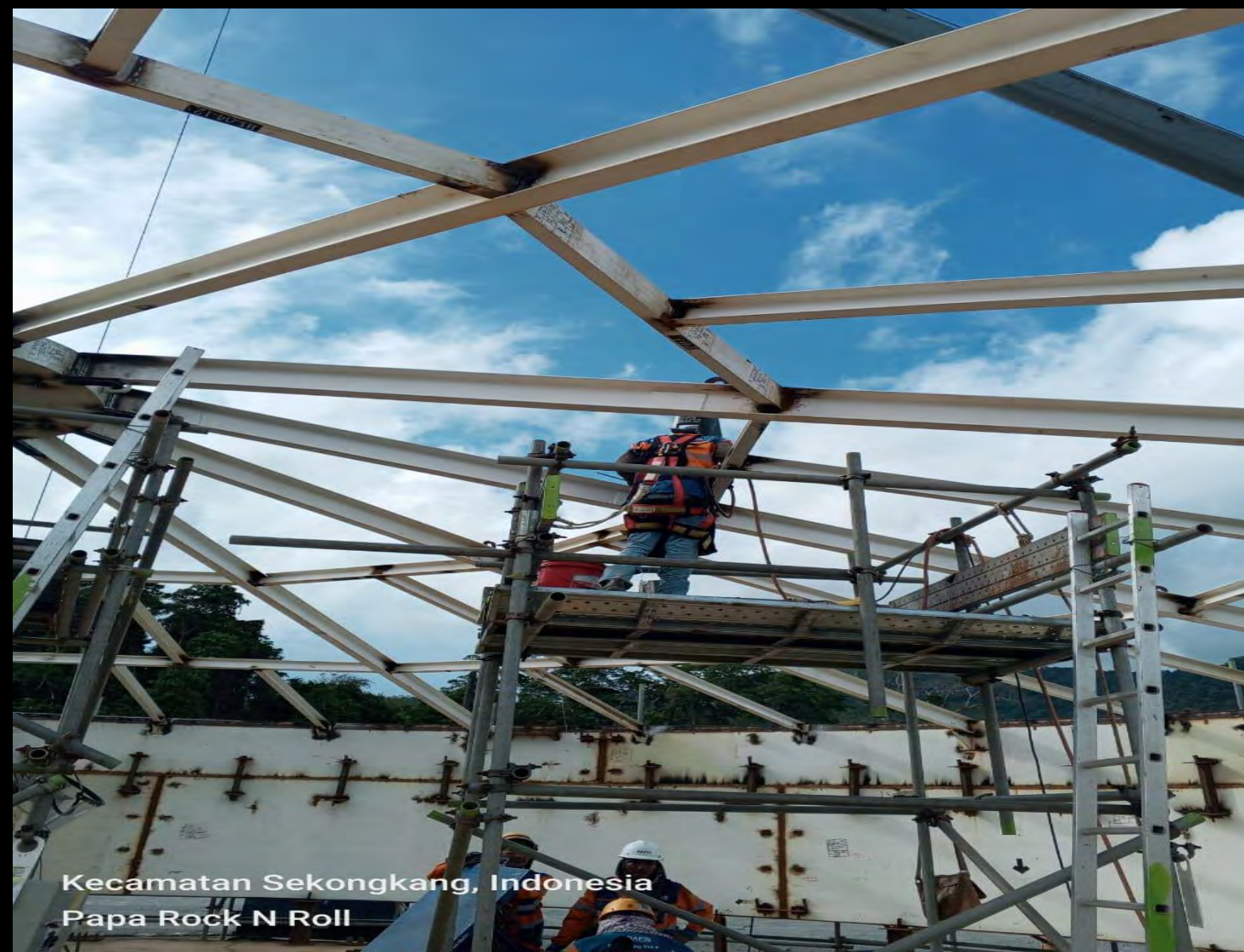
INSTALATION OF RAFTER WATER TANK
