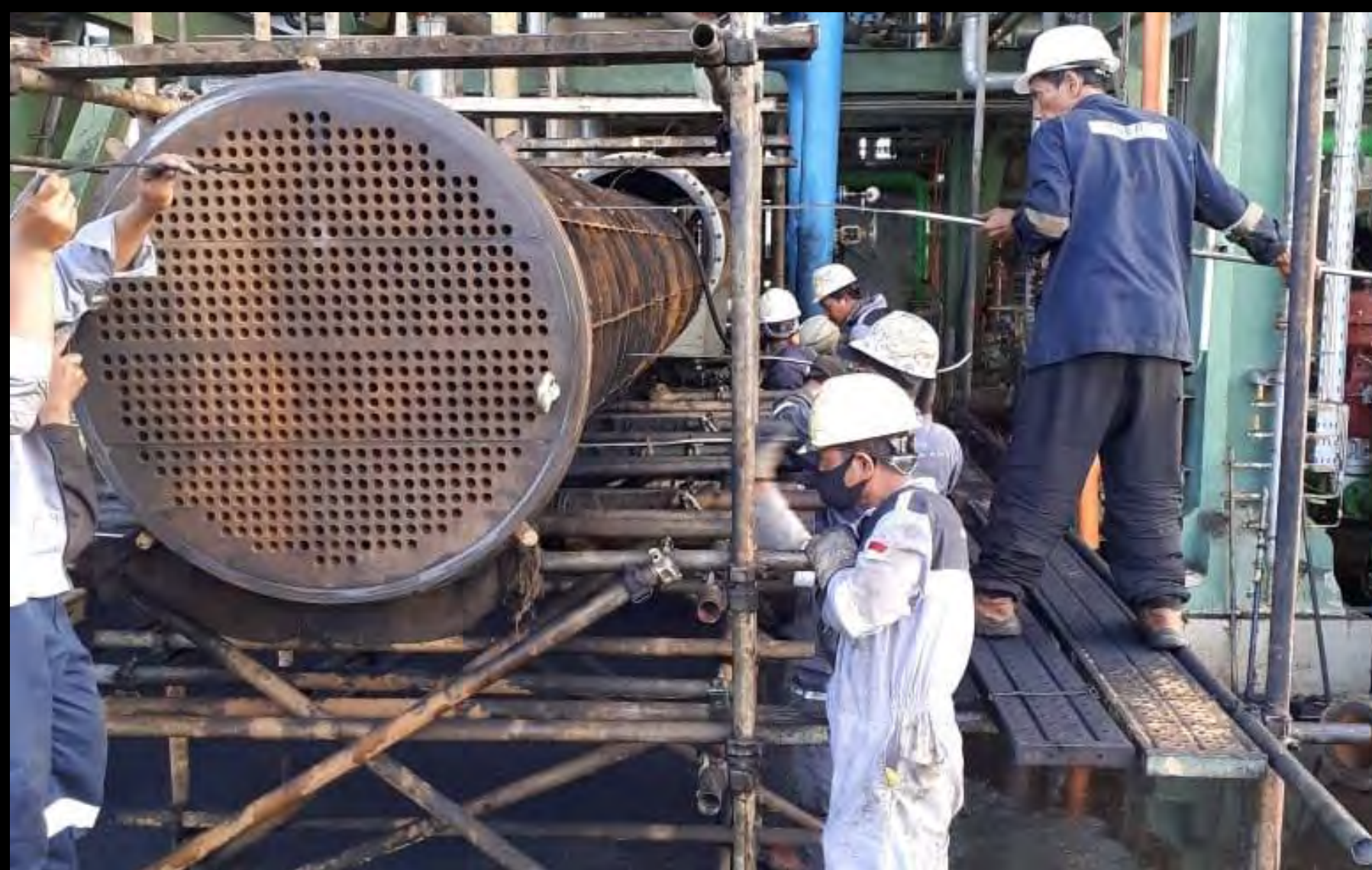
HEAT EXCHANGER (HE) DISASSAMBLING
