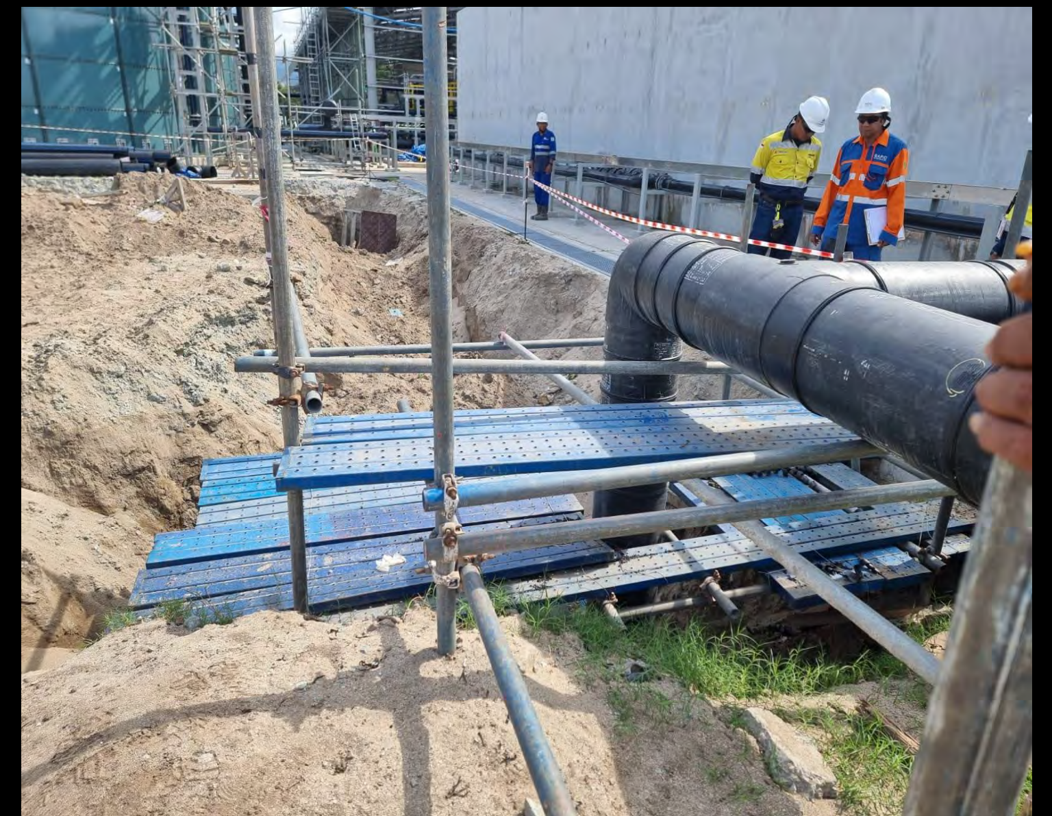
SEA WATER UNDERGROUND PIPELINE
