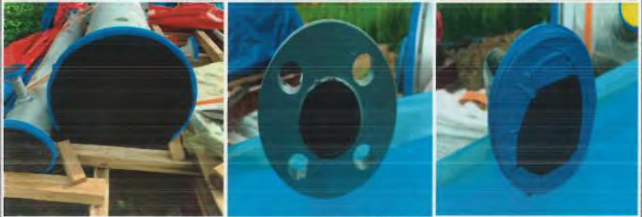
Preservation Cleaning, Apply Vpci 368, Vpci 137, Apply Rubber & Covering For Spool & Valve
