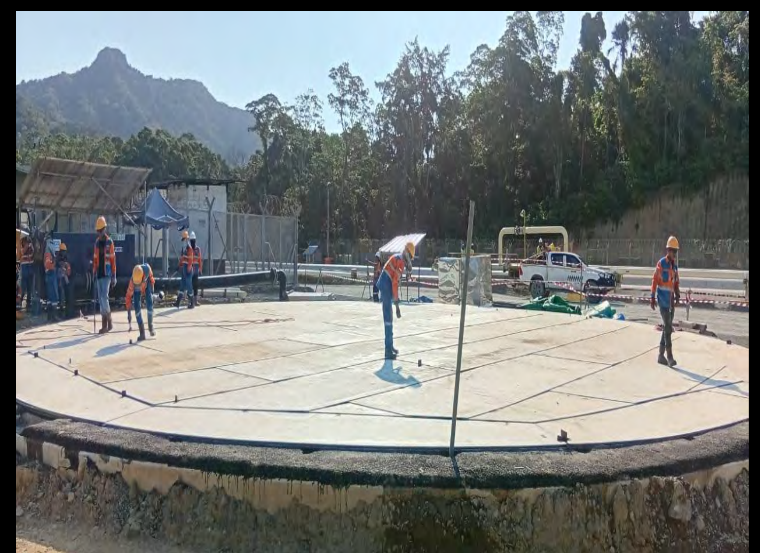
LAYING BOTTOM PLATE & ANNULAR PLATE WATER TANK
