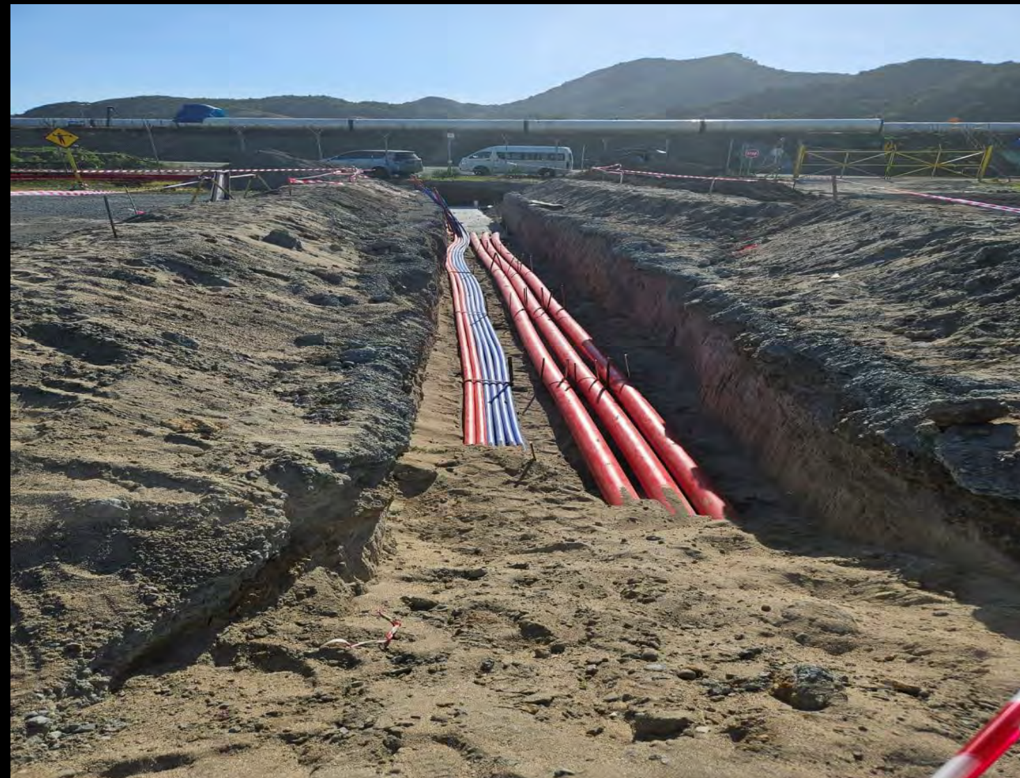
UNDERGROUND CABLE POWER AND FIBER OPTIC USE HDPE CASING
