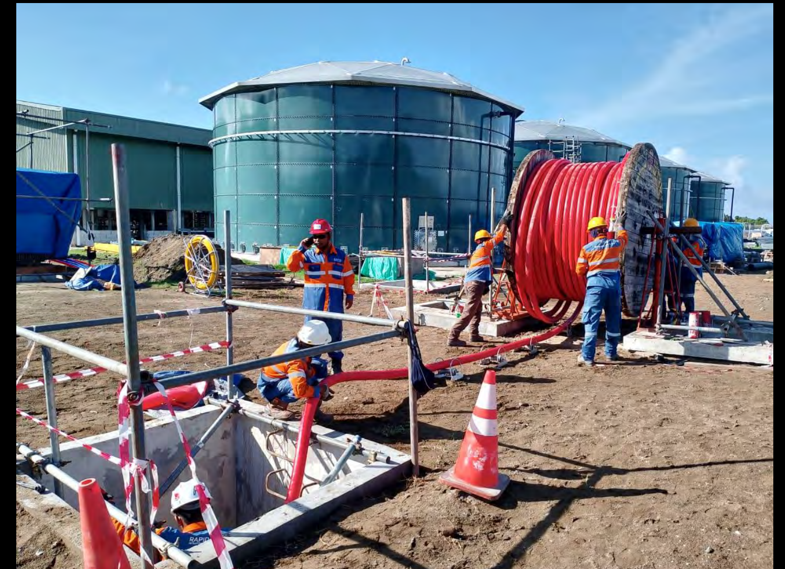
PULLING OF POWER CABLE ACTIVITY
