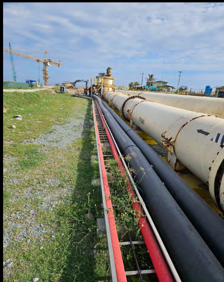
SEA WATER 14" & BRINE 12" ABOVE GROUND PIPELINE
