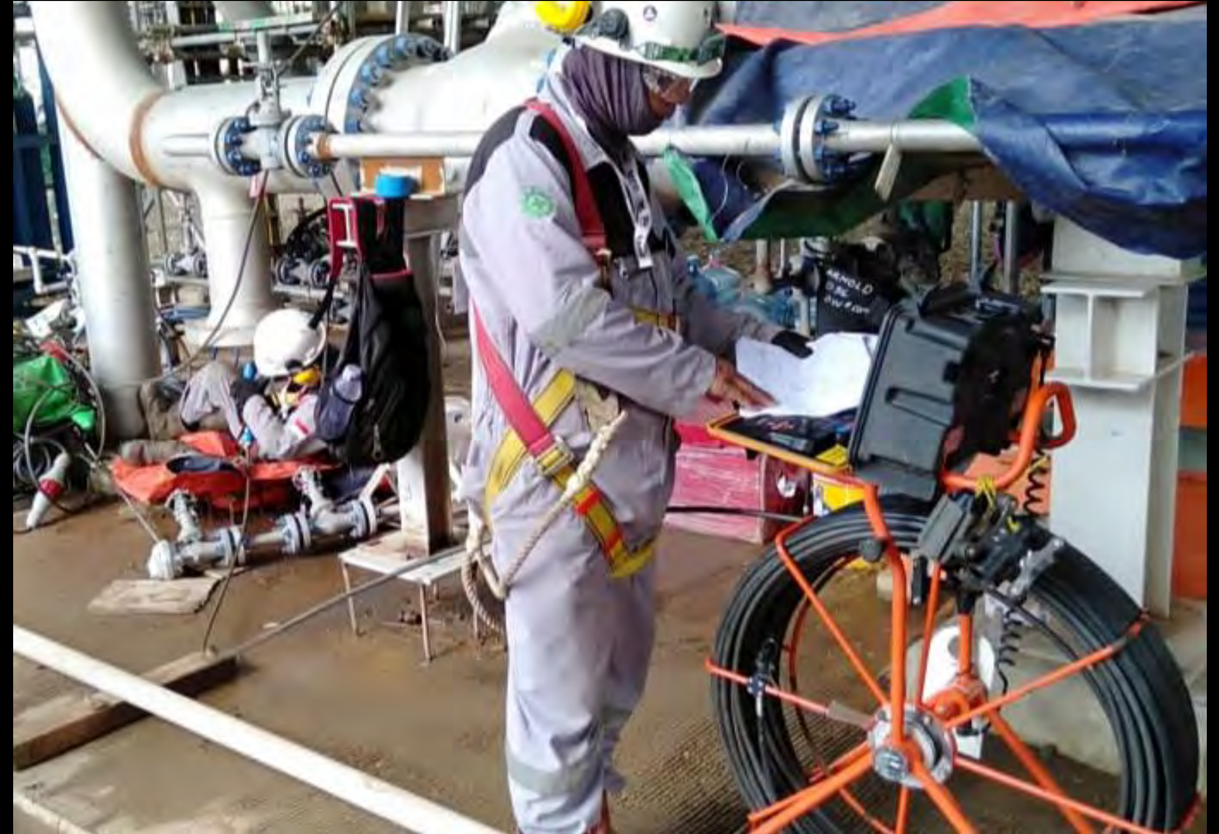
INSPECTING PIPE THROUGH MONITOR USING FLEXIBLE BORESCOPE
