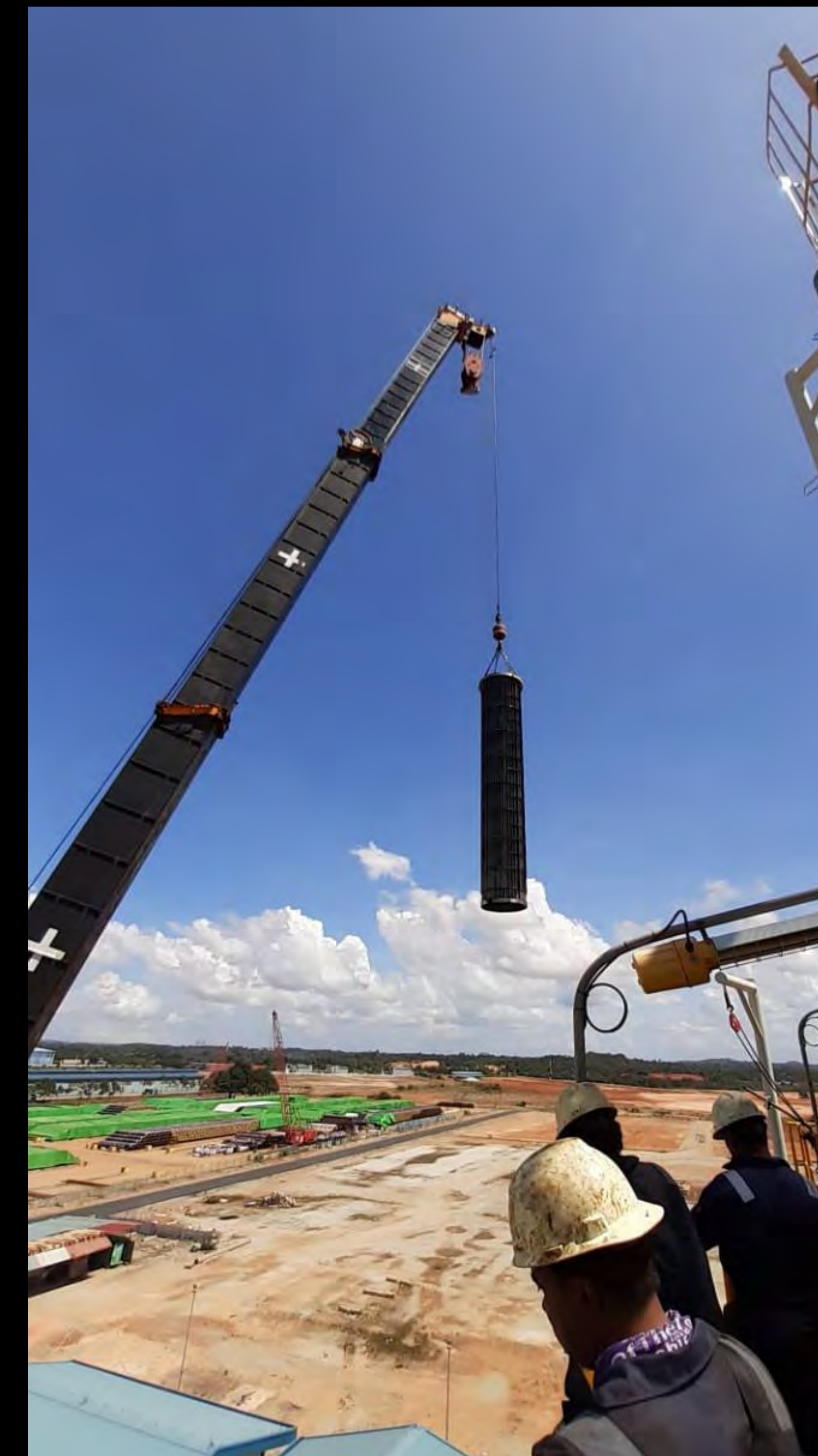
HEAT EXCHANGER TUBING LIFTED
