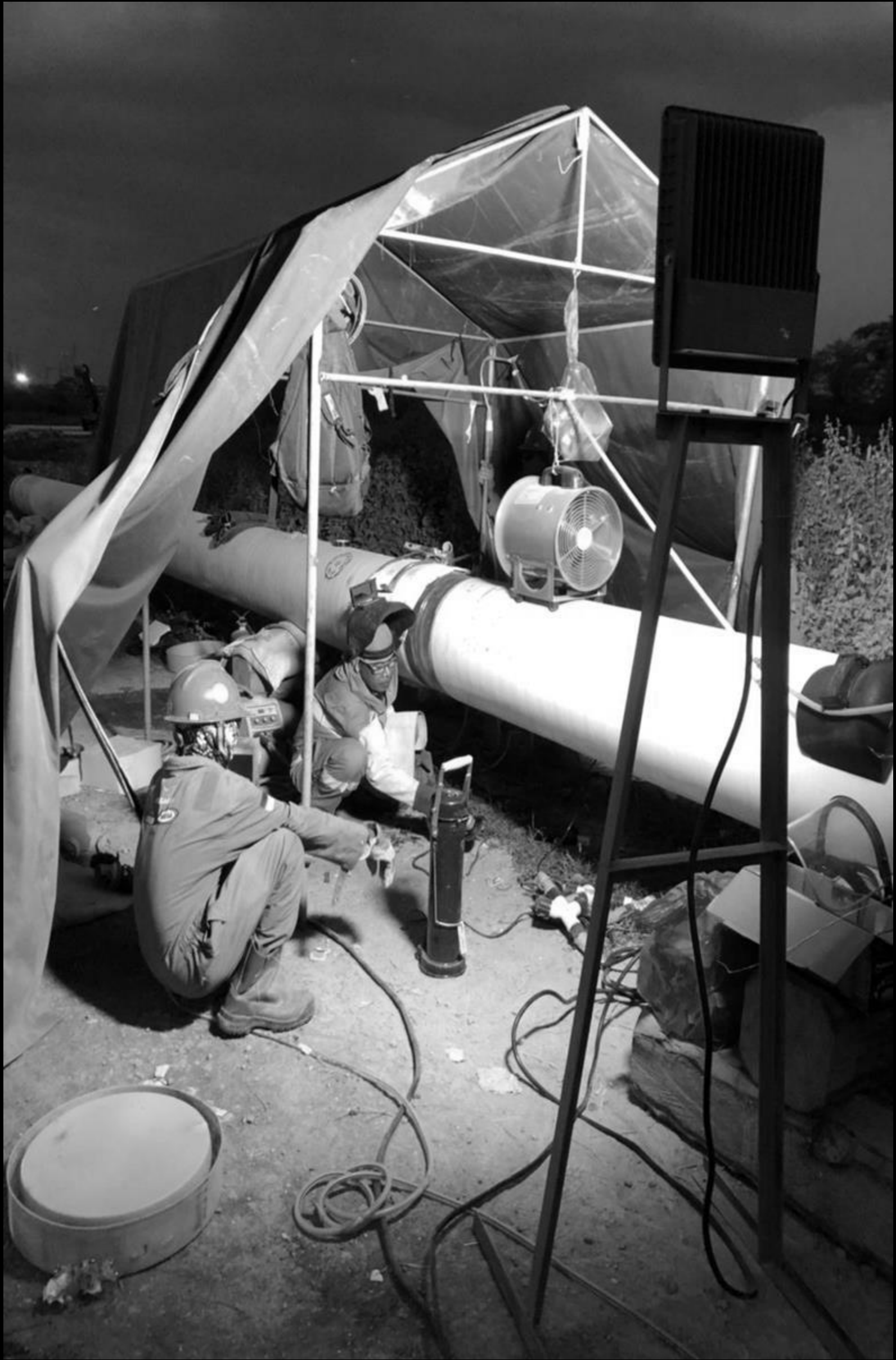
WELD INSPECTION
