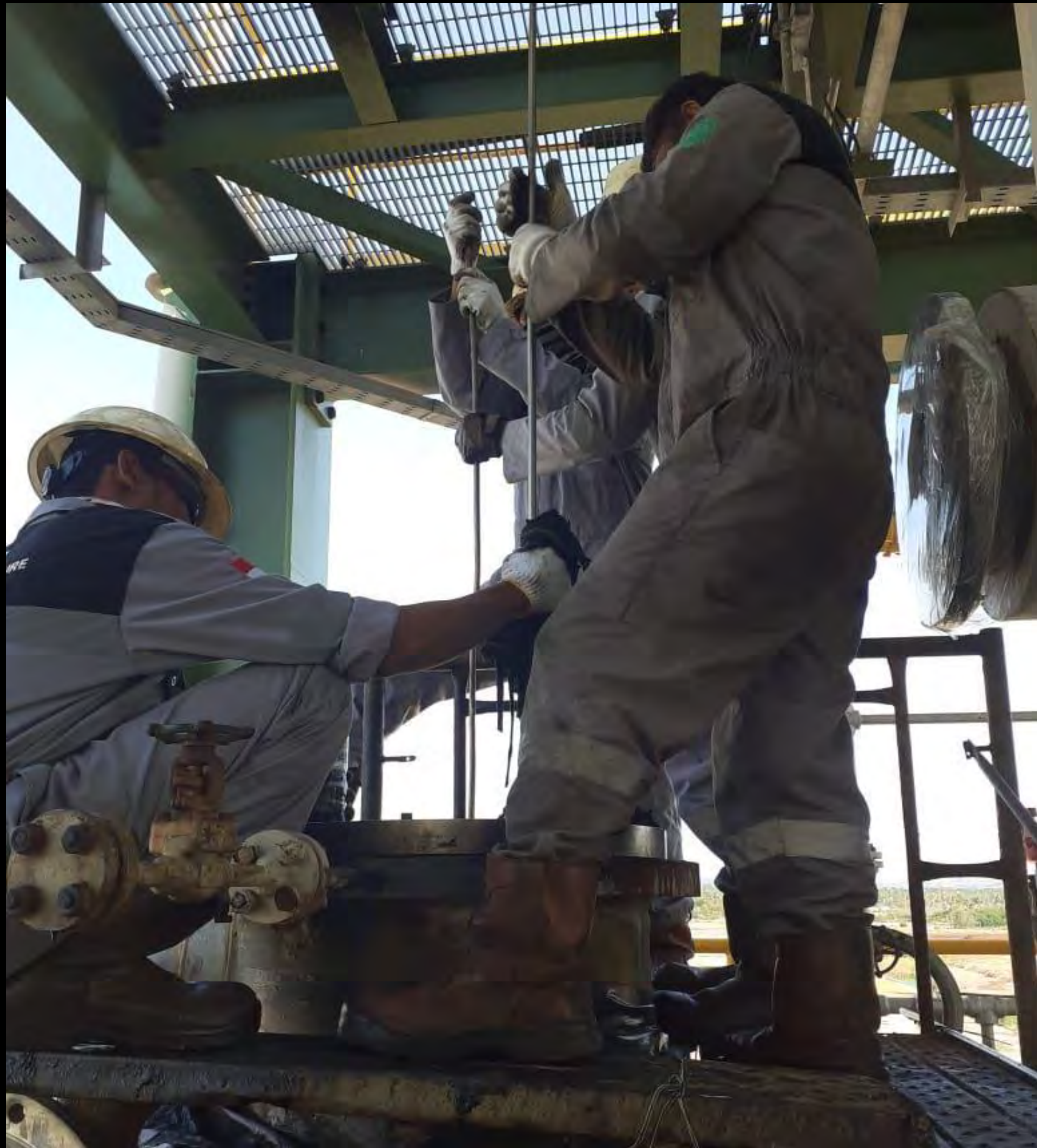
HEAT EXCHANGER CLEANING
