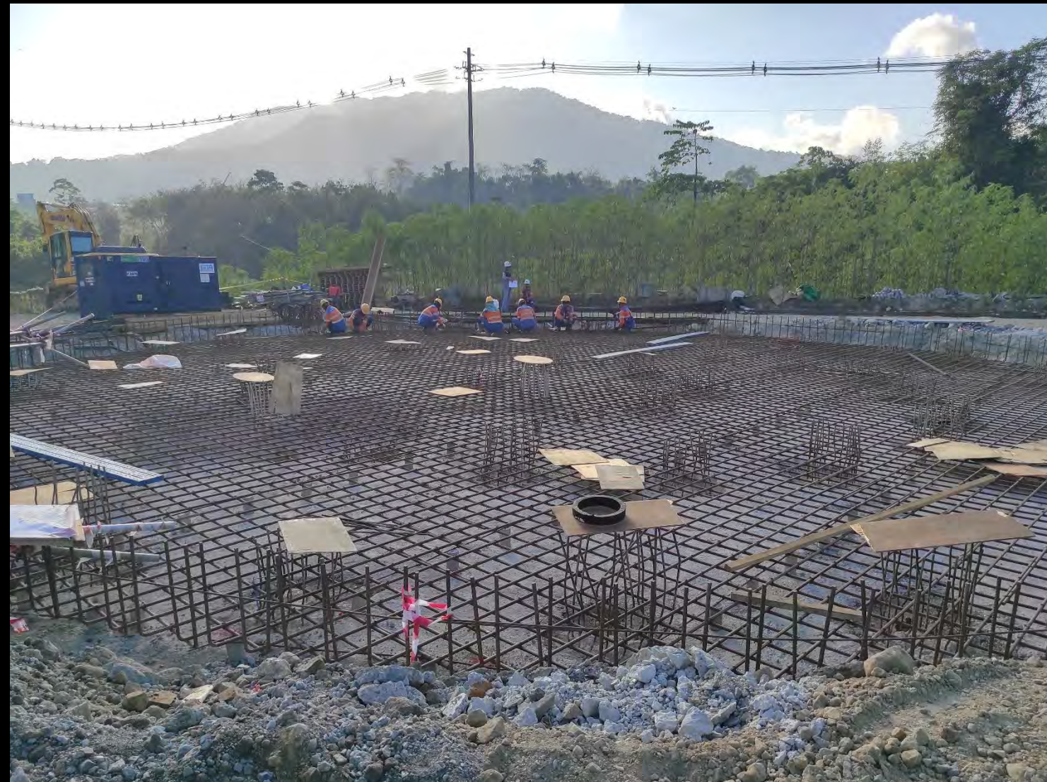
INSTALLATION OF REBAR
