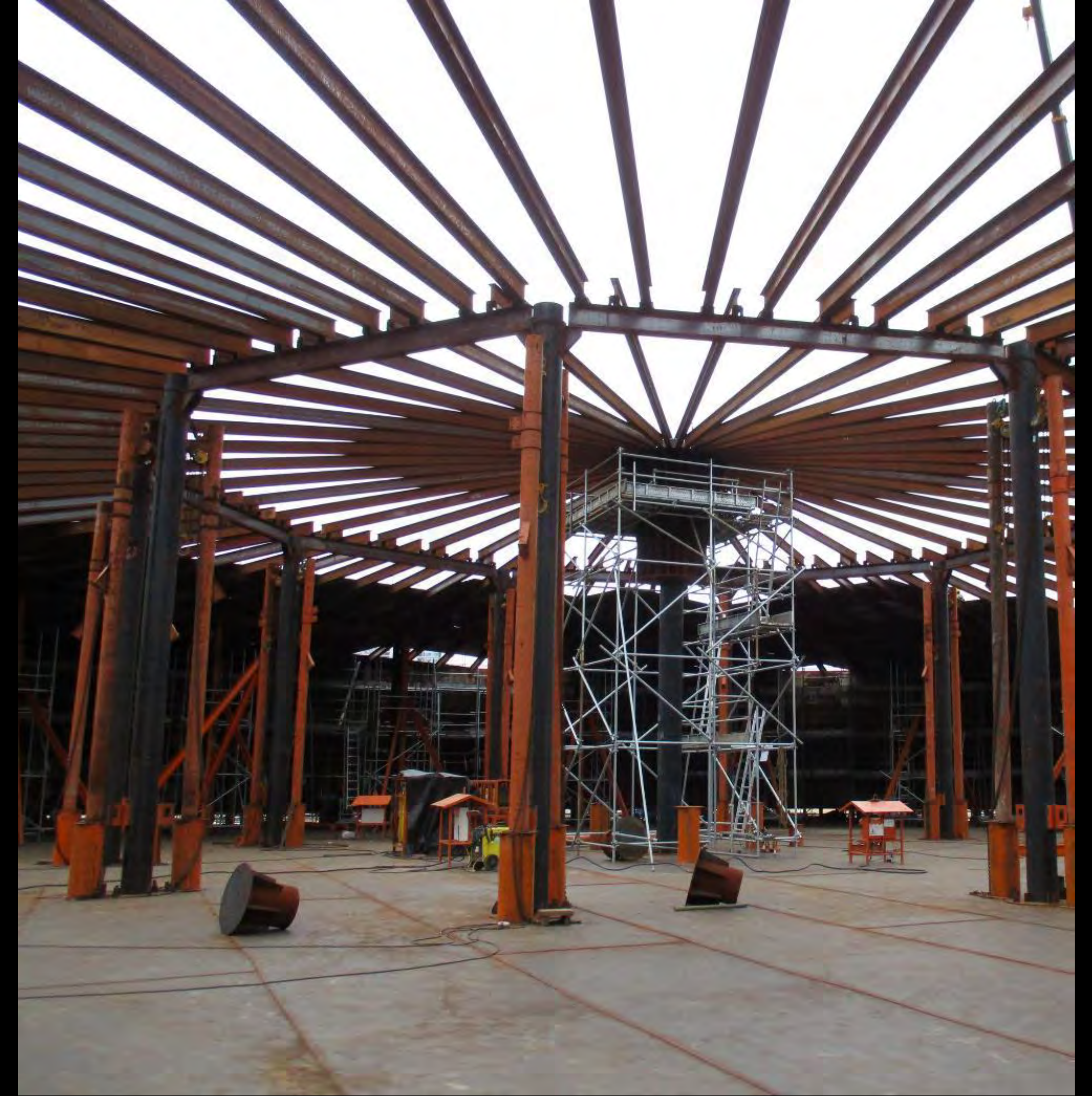
INSIDE VIEW OF CRUDE OIL TANK
